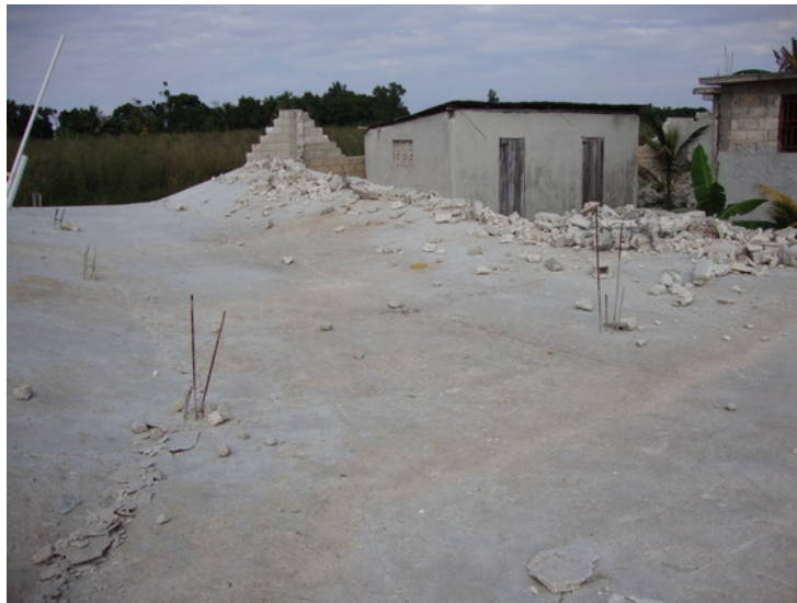
Figure 4.12. Strong Consensus Type 2: Building entirely collapsed.
